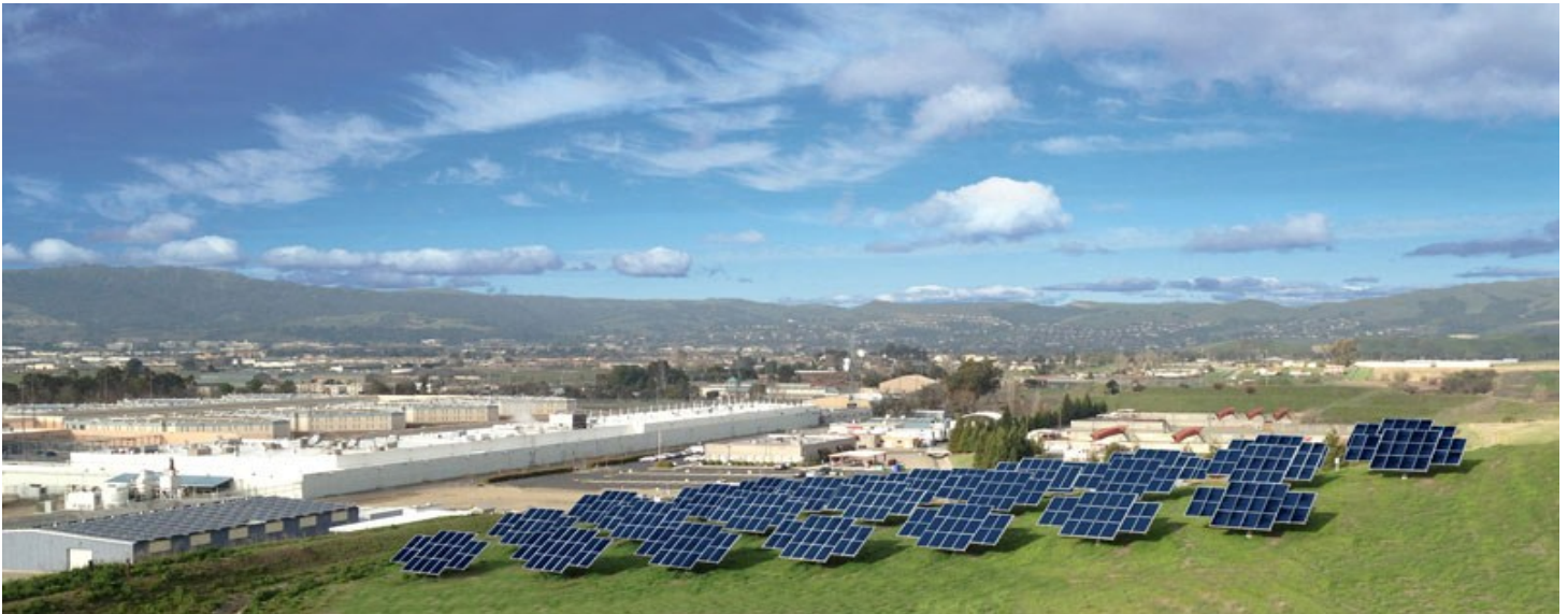
Solar Panels at Santa Rita Jail, Alameda County
